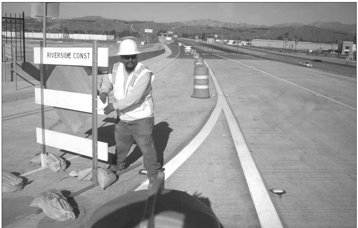
FINAL LINK IN MISSION BOULEVARD OVERPASS AT SR 71 OPEN FOR BUSINESS – Officials from Caltrans, Pomona's Department of Public Works and several contractor crews moved the barriers, changed the signs and opened the last two on and off ramps for business this month at the Mission Boulevard overpass at State Route 71. The southbound off ramp and the northbound on ramp were opened – this time without ceremony – to full traffic. The bridge, the southbound on ramp and the northbound off ramp all were opened in August with full ceremony and numerous elected officials and city and state personnel on hand. Pomona Mayor Elliott Rothman called the project "the single largest public works project in Pomona's history." It was the key element in a $40 million grade separation project. Pictured working on opening day on the new southbound off ramp (looking north) is Jeff Quiroz, of Alcorn Fence Co. in Riverside.
