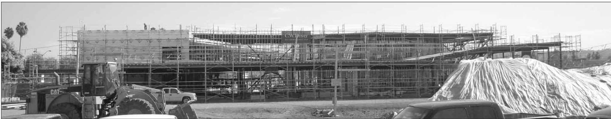
NEW IPOLY BUILDING NEARS COMPLETION, OPENING EXPECTED THIS FALL – Progress is well under way for the new iPoly High School building on the Cal Poly Pomona campus where the new structure will replace the modular units that have served as the home of the school since it opened in 1993. Students beginning in the fall will be the first to use the new $20 million school site. The school, which partners with Cal Poly, serves 500 students from more than 40 cities. The specialty high school, built on a charter school model, is a tuition-free high school that focuses on hands-on project-based learning.
