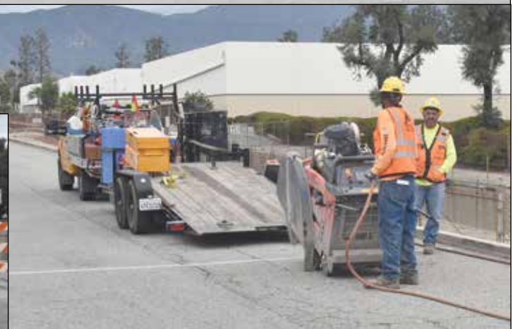
Workers roll out a concrete cutter to go to work on relocating utilities in preparation for a new Foothill Gold Line crossing at Fulton Road just west of the North Pomona train station on Feb. 1, the first day of a 90-day road closure at the site. Pictured is a look to the north from just north of the existing tracks.
