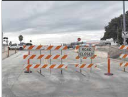
Here's a photo looking south on Fulton Road with the existing tracks in the background.
