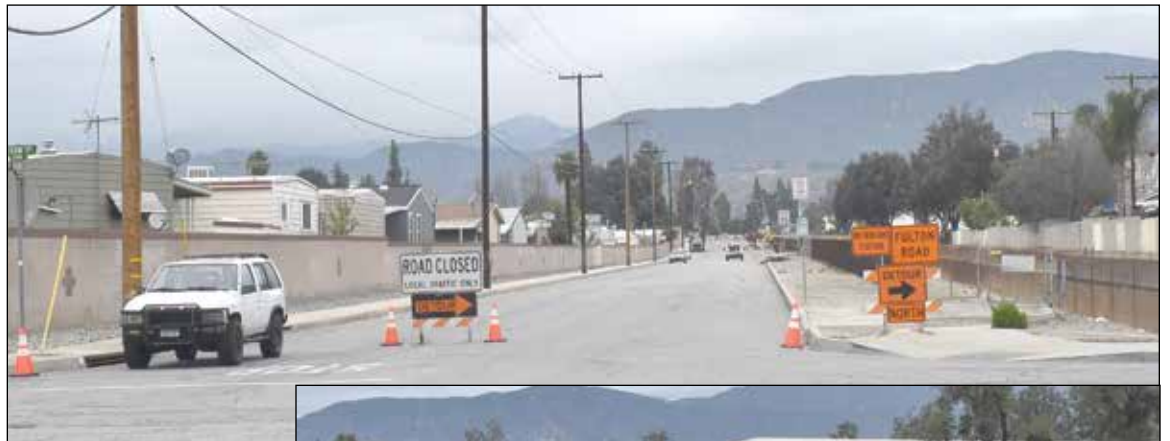
Pictured is the new road closure for Foothill Gold Line construction looking north on Fulton Road from Arrow Highway.
