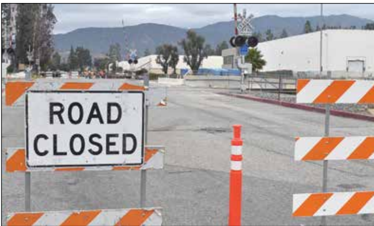
Photo shows Fulton Road looking north from just south of the existing tracks.
