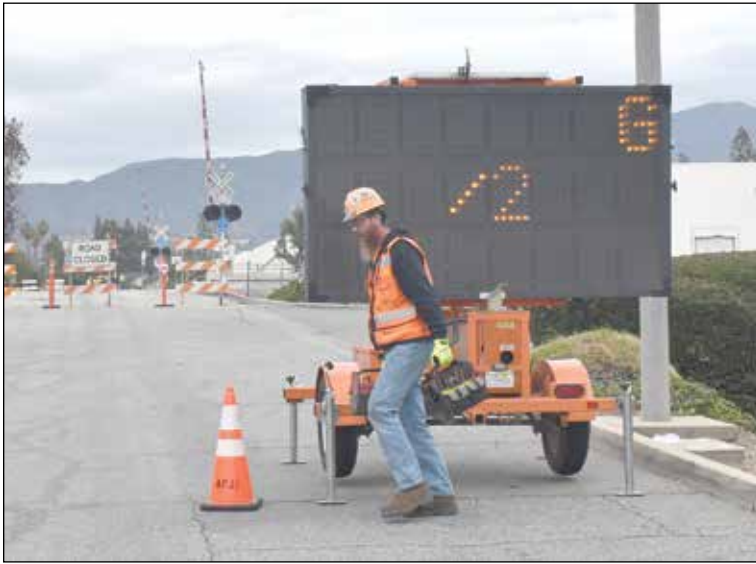
A worker with contractor Kiewit-Parsons sets up a road closure information sign in the northbound lane of Fulton Road on Feb. 1, the first day of the first road closure in Pomona due to the Gold Line construction project into the future North Pomona Gold Line station, which will be located just a couple of hundred yards to the east.
