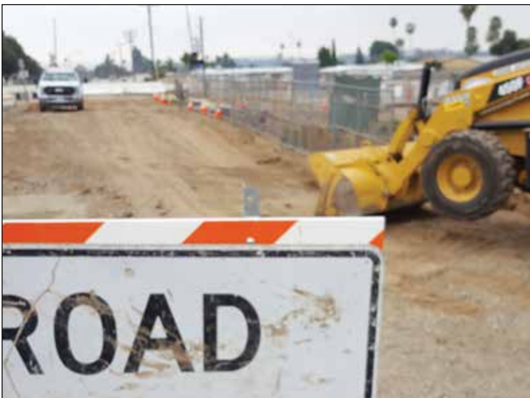
A week after the road closure, work crews were well under way with pavement removed and trenches dug for pipe relocation. Pictured is Fulton Road looking south with the tracks in the background.
