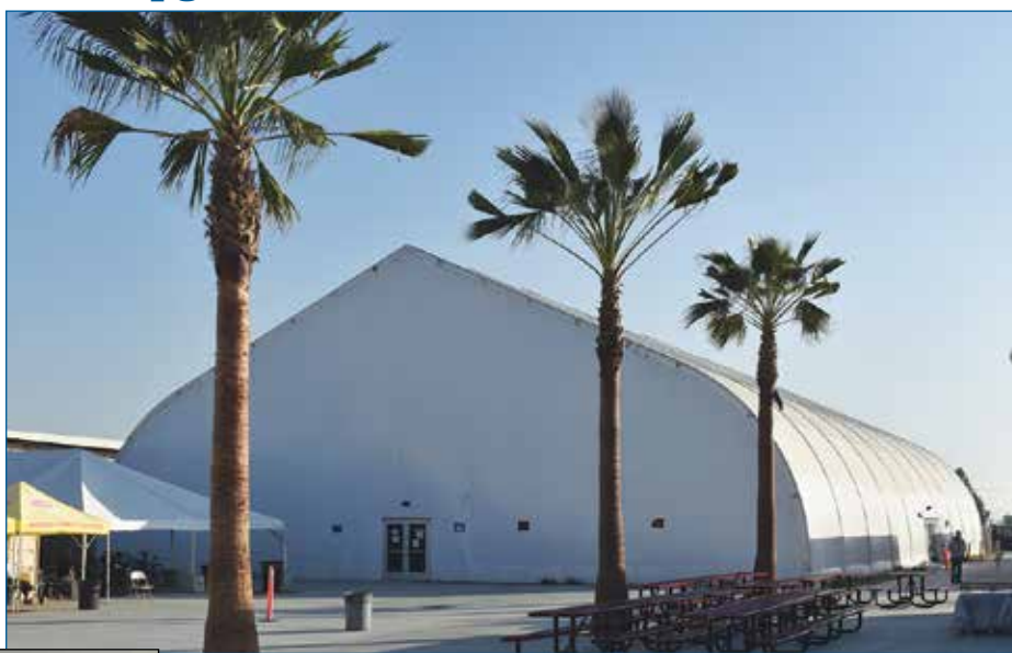
The huge tent-like structure housing sleeping quarters, a dining area and other facilities has been open for business for the past year at 1400 E. Mission Blvd., Pomona, on the site of a former Yellow Cab dispatching center.
