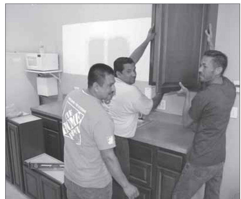
FINISHING TOUCHES AT HOUSE OF RUTH -- Volunteers from Home Depot stores in Pomona, Chino and Rancho Cucamonga install new cabinets this month in the kitchen at Pomona's House of Ruth. About 40 volunteers -- 10 from House of Ruth and the rest from Home Depot -- spent a full week working on a facelift valued at nearly $40,000 including painting, laying flagstone, installing new blinds and installing the kitchen cabinets. Actual supplies were made possible through a Home Depot Foundation grant. Pictured, from left, are Adrian Reynoso, George Estrada and Craig Timentel, all of the Rancho Cucamonga Home Depot store.
