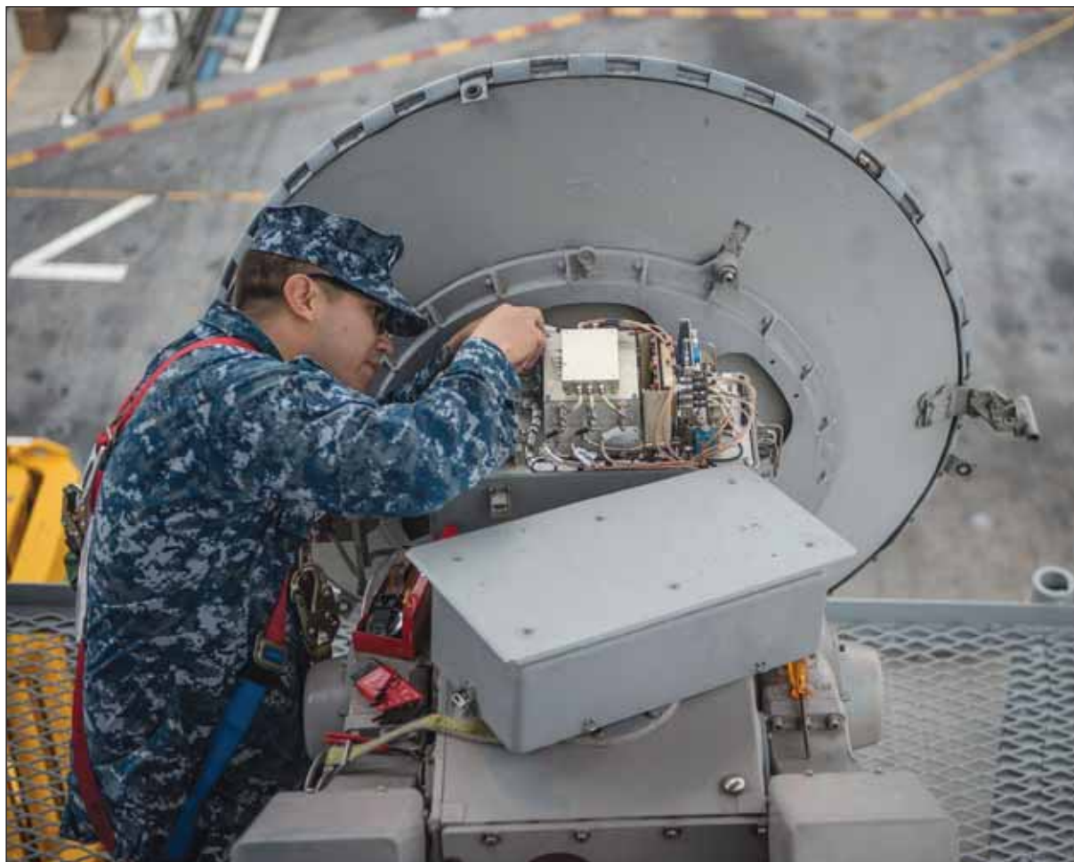
Photo courtesy of Navy Mass Communication Specialist 3rd Class Cody Hendrix POMONA NATIVE WORKS ABOARD USS RONALD REAGAN -- Electronics Technician 3rd Class Diego Martinez, a native of Pomona, installs a power monitor in an SPN-46 radar aboard the aircraft carrier USS Ronald Reagan (CVN 76). The aircraft carrier is homeported in San Diego at Naval Base Coronado.
