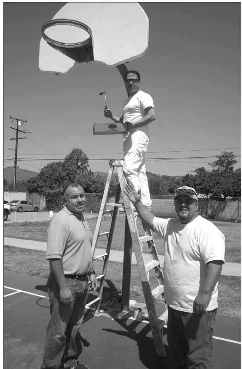
PAINTING THE BASKETBALL BACKBOARDS -- Luis Rodriguez of Whittier, of Mayans Development in Yorba Linda, pauses on the ladder for the camera as he adds a new coat of paint to a basketball backboard at Pomona's John F. Kennedy Park during the "Community Helping Hands Service Project," a major clean-up effort. Pictured on the ground, from left, are Pomona City Councilman Freddie Rodriguez and Pomona Parks and Recreation Commissioner Carlos Goytia, an organizer of the event and also a board member representing south Pomona at Three Valleys Municipal Water District. "It's inspiring and humbling and exciting," said Pomona City Councilman John Nolte, an organizer of the event, adding that it "shows what we can do when we get the city, community churches and families together." A skip loader was even on the job for the baseball field part of the project, courtesy of Chuck Clark's 3D Service of Pomona.
